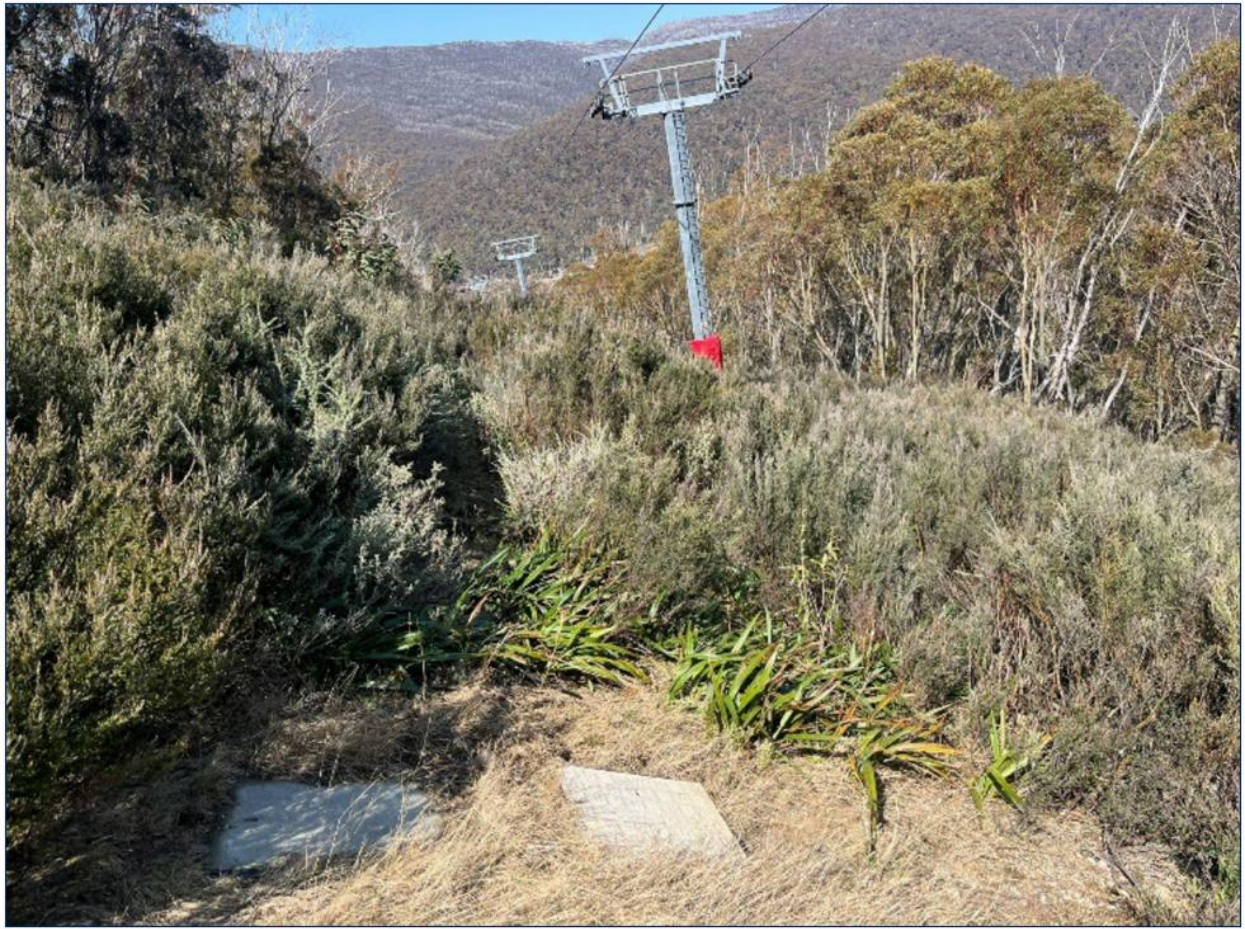
Figure 4 | Location of Gunbarrel Chairlift tower 12 which will support the proposed lift camera (Source: Applicant's Statement of Environmental Effects [SEE] 2024))
